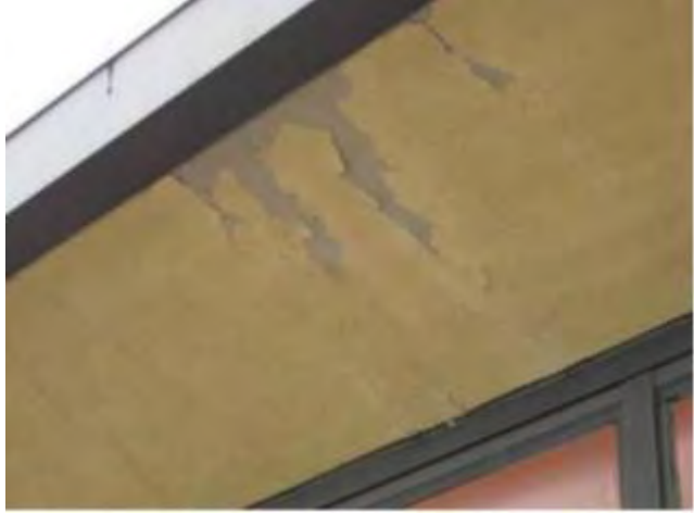
Soffit deterioration
