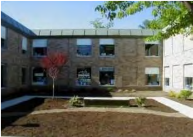
Original single pane windows
